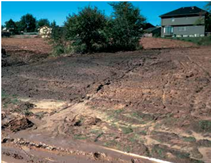
In this suburban neighborhood, sediments were washed into the street by the rain, because the soil was not protected during house construction.
