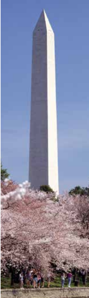
The outside of the Washington Monument in Washington, D.C. is made from white marble from the state of Maryland.
