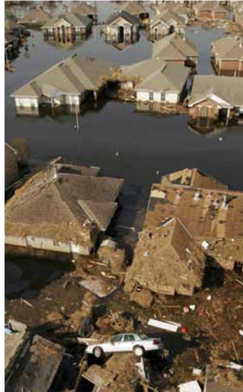
After Hurricane Katrina passed through New Orleans in 2005, flood waters caused even more destruction and forced a complete evacuation of the city.
